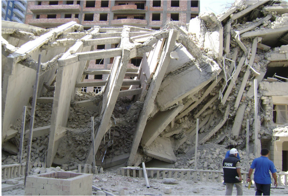
Figure 1. Suddenly Collapsed Building in Baku, 2007.
