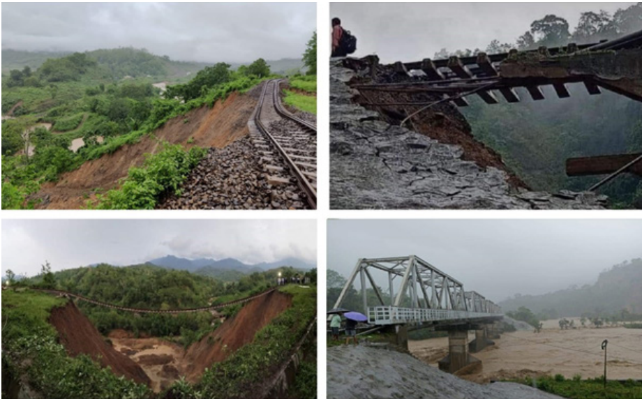
Fig 1C: Specimen photographs of eroded section of railway line along the Maibong and Ditokcherra stretch (Sources: ASDMA).
