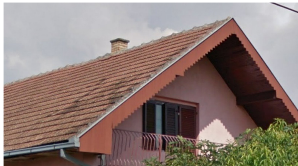
Figure 6. Entirely closed roof without any hollow places between walls and roof. Google Street Imagery 2014.
