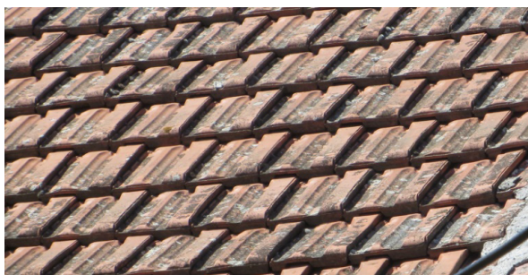
Figure 20. Regular roof tiles.
