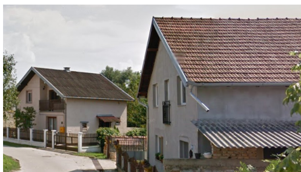
Figure 21. Houses with two floors and a gable roof type. Houses with two, three, or more floors will have a greater probability of suffering damage during windstorm events. Google Street Imagery 2014.
