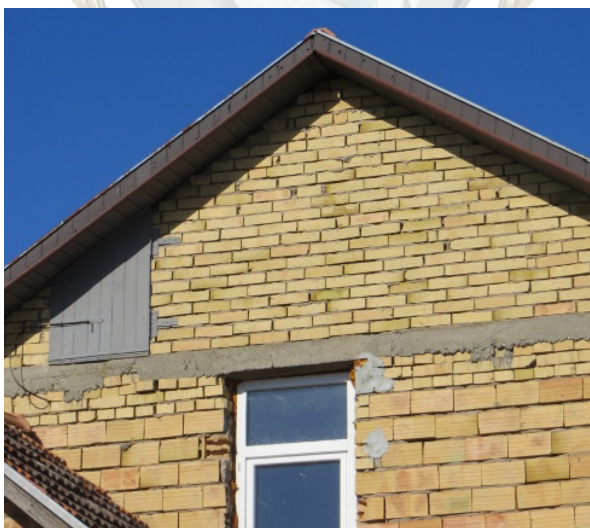
Figure 22. Polyvinyl Chloride (PVC) door and window with double glass and a metal door with good holders on the sides. Roof sides with two brick rows with plaster as bonding material, with reinforced brick supporting pillars. This type of roof side is highly resistant to damage from windstorm events.
