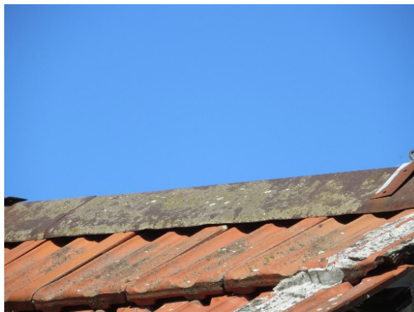
Figure 7. Metal roof ridges are tightened to the roof tiles. This is one of the most exposed and vulnerable parts of the roof during a windstorm event.
