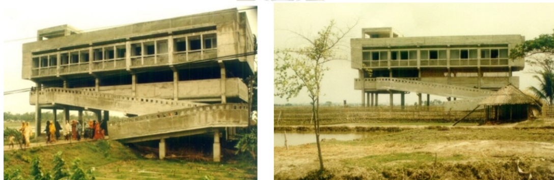
Figure 4. Cyclone Shelter PRISM (Photo: Bashirul Haq and Associates)
