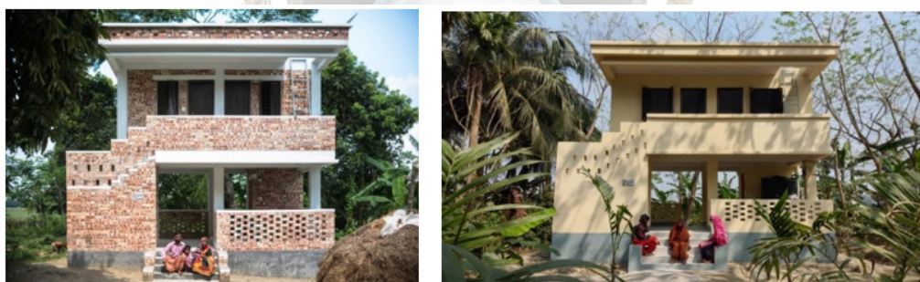
Figure 15. A Cyclone Resilient House by BRAC (Photo: Ashraful Haque)
