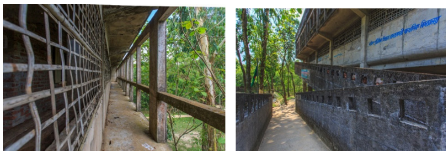
Figure 16b. Existing condition of PRISM Cyclone Shelter (Photo: Author)
