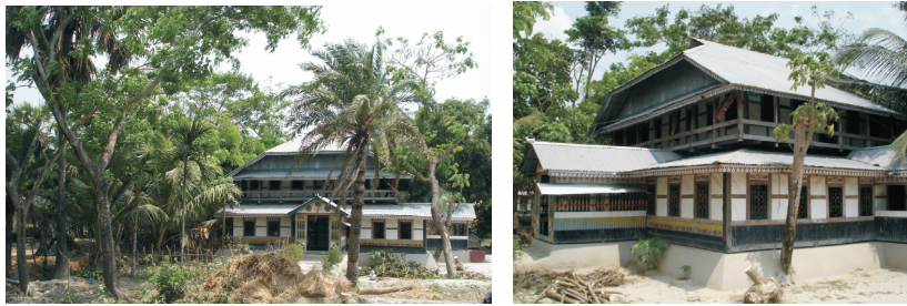
Figure 21. an indigenous Disaster Resilient House in a coastal area. (Source: Bashjirul Haq and Associates)
