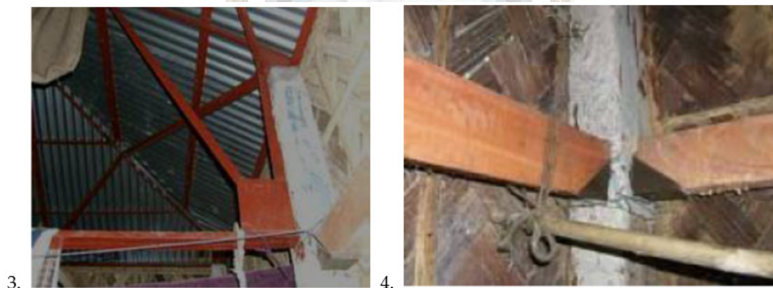
Figure 18. 3 & 4 Improved connections of R.C.C. pillars with steel roof (Source: Shelter Cluster)
