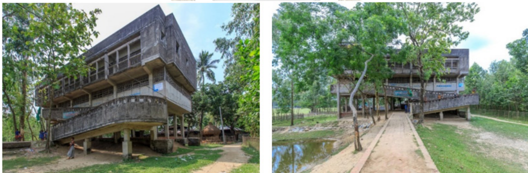
Figure 16a. Existing condition of PRISM Cyclone Shelter (Photo: Author)
